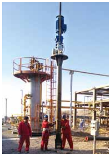
Vertical pump being installed
