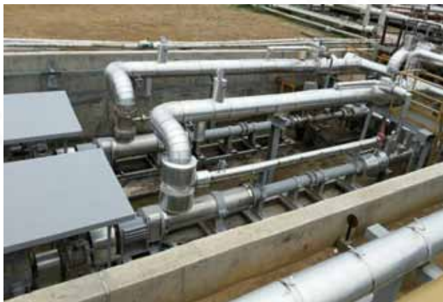
Two sets of pump being installed in parallel in Indian oil field
