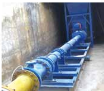
Pump for Mud Cake Transportation Installed before Incinerator
