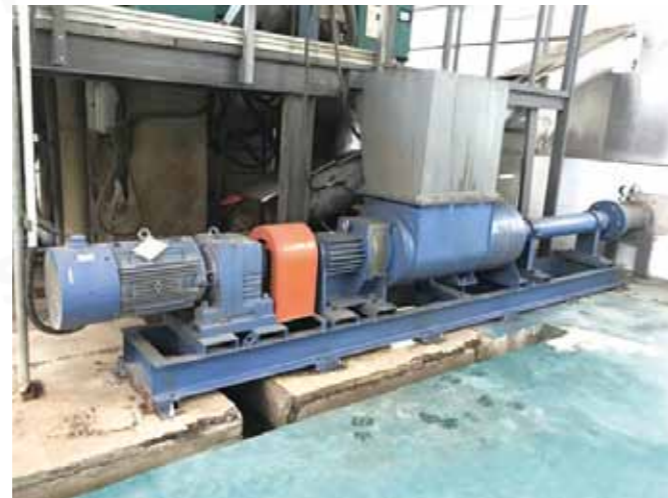
M2 class hopper pump to transfer mud cake 18%-20% solid content
