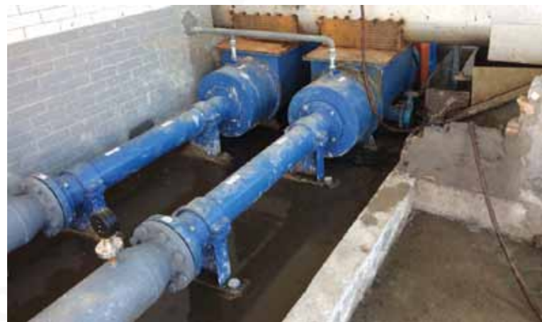
Open throat hopper pump to transfer mud cake 20-25% solid content
