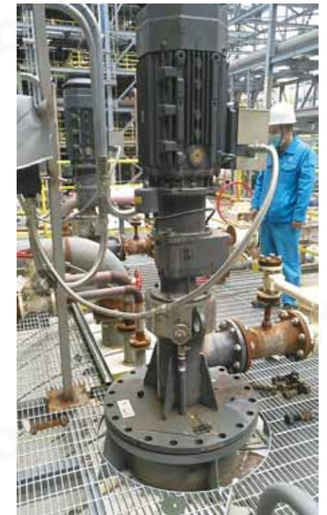
Subtor vertical pc pump used for chemical sewage transportation
