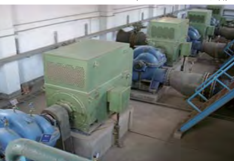
↑ 河北峰峰集团薛村矿电厂 (SLOW 200-530(I)AT, 4台) Hebei Fengfeng Group Xue Village Mineral Power Plant
