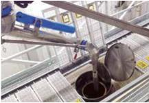
shut-off valve. These are mounted on standposts at gantry floor level and can service 2-3 manhole openings on a correctly positioned tanker.
